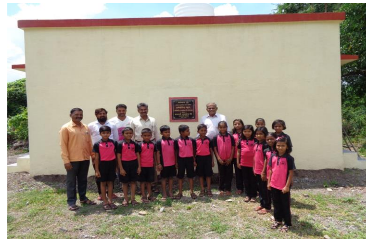
Constructed 2 Class Room At Lokseva Secondary & Higher Secondary School, Agalgaondt.
